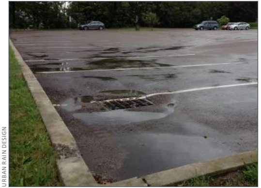
▲ EXISTING: A typical oversized parking lot stall in Vermont.
