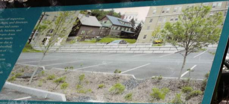
Stormwater runoff in a parking lot at 133 State Street captures and treats stormwater runoff. Credit: Vermont Department of Buildings & General Services.
