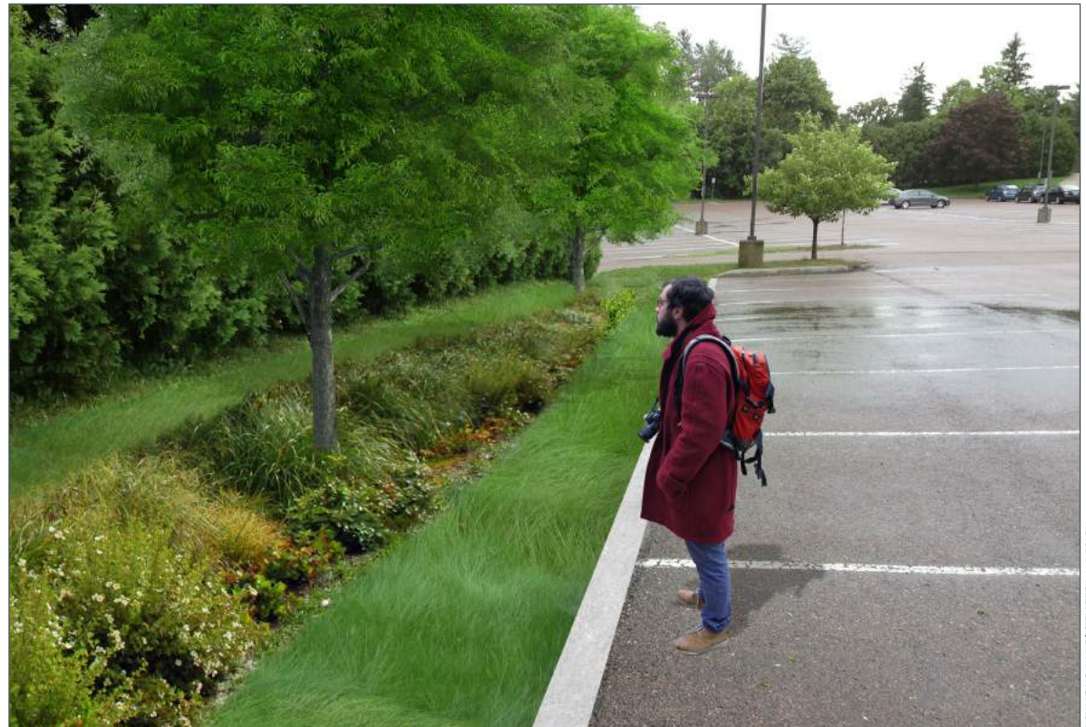
▲ RETROFIT OPPORTUNITY: The same parking lot perimeter space retrofitted with a vegetated swale. Notice the amount of plant diversity compared to just a mowed lawn space.
