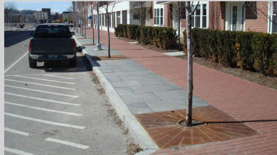
▲ These street trees are installed with structural soil to increase soil volume and allow for greater root expansion. (Winooski)
