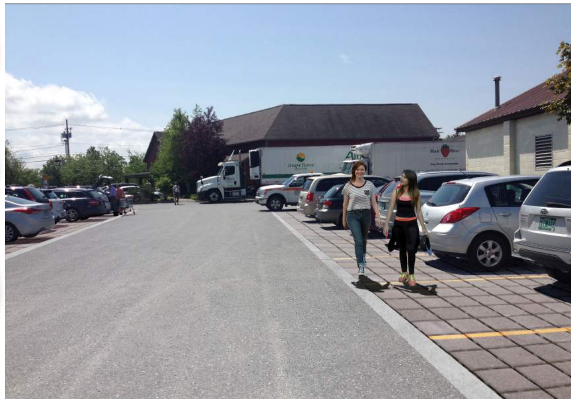
▲ RETROFIT OPPORTUNITY: The same parking lot retrofitted with pervious interlocking concrete pavers within the parking stalls.
