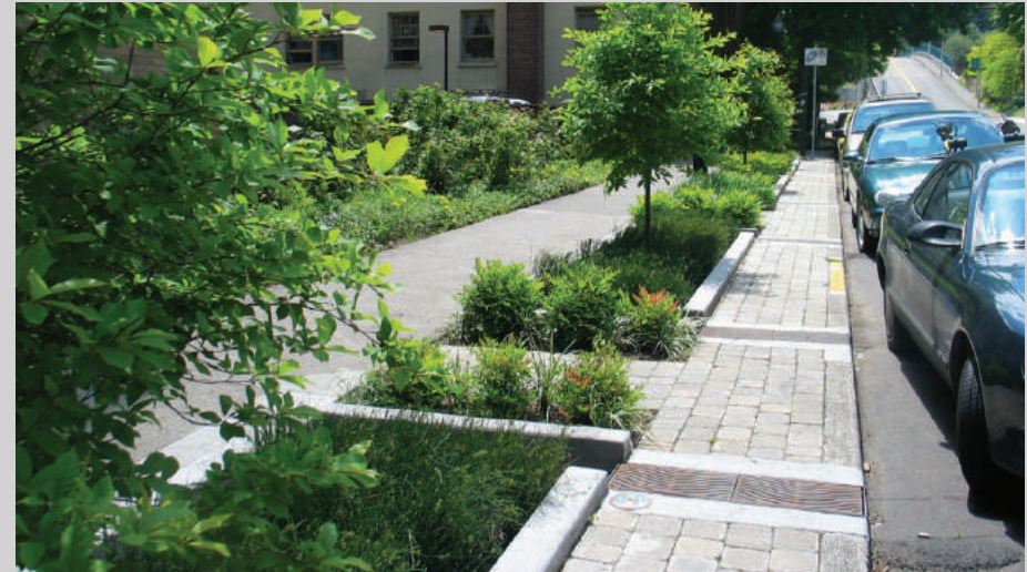
▲ This Green Street project utilizes a series of stormwater planters while maintaining on-street parking and adequate space for pedestrian circulation.
