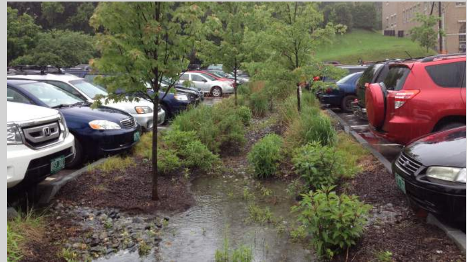
▲ Green Streets captures runoff and pollutants and treats it prior to entering a nearby creek, stream, river, or lake. (Montpelier, VT)
