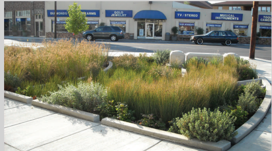
▲ This street rain garden has two planting zones with dry-tolerant plants placed on the side slopes and wet-tolerant plants placed at the lowest elevations..
