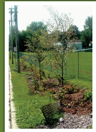
Trees enhance bioretention areas and add aesthetic value. Burlington, VT.
