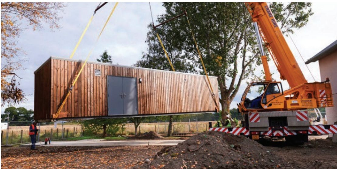
FIGURE 5: Installation of a containerized system
