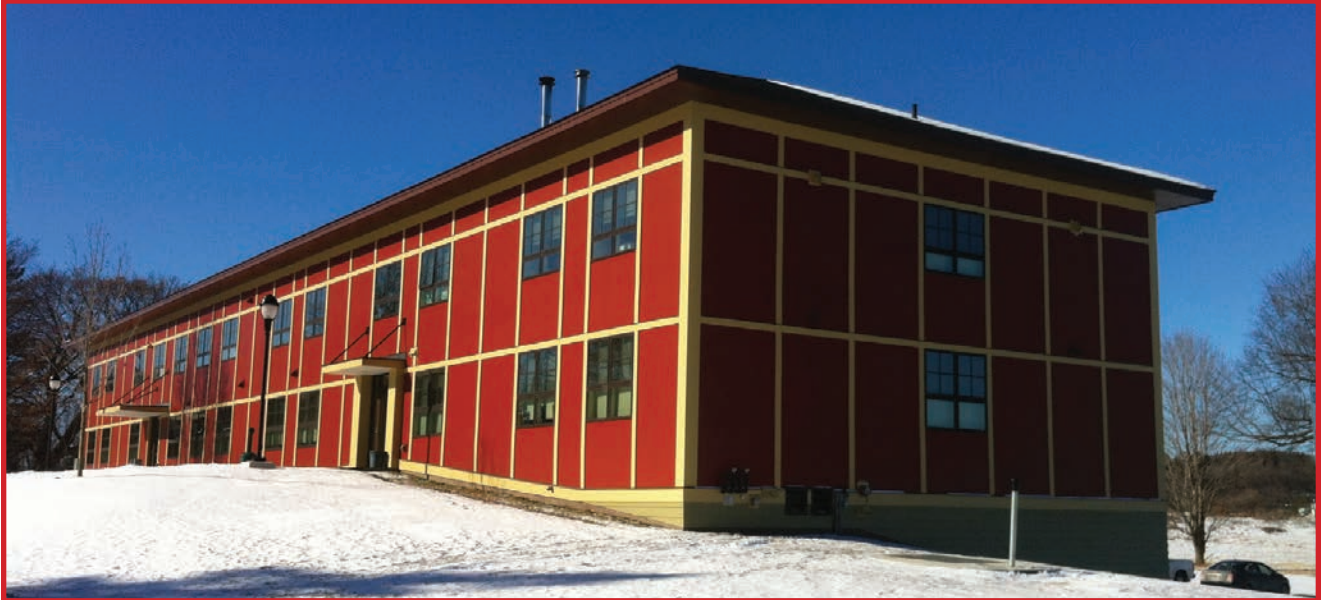
Courtesy/ Biomass Energy Resource Center
