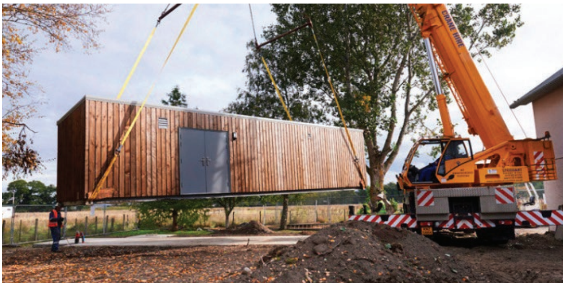
FIGURE 5 Installation of a containerized system
